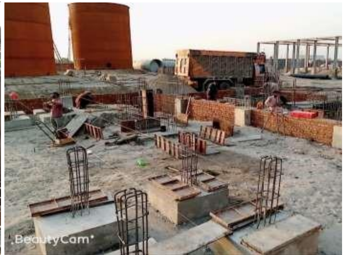
246-Construction of Foundation of Boiler
