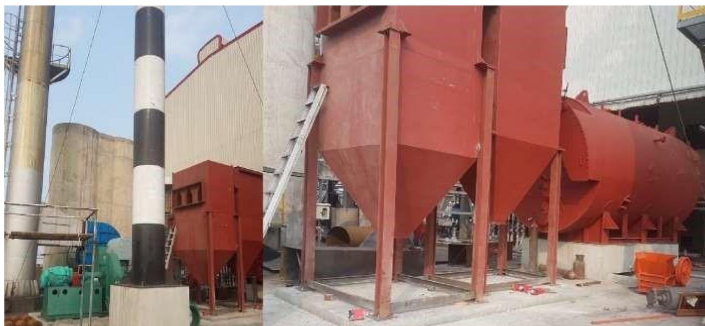
231- Foundations of Boiler Multi Cyclone, Chimney, Hooper Machine & Stairs
