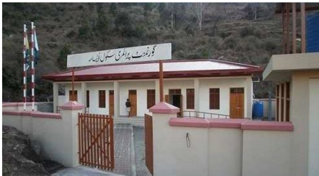
102-Completed Picture of GPS Atisa, UC Danna, District Muzaffarabad, AJK
