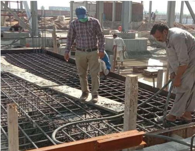
246-Raft Foundation of HT Oil Heater
