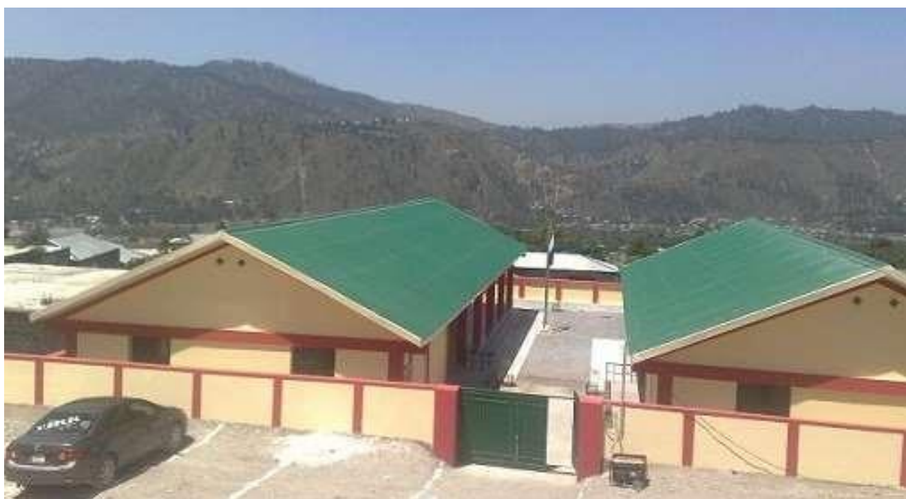
103-Completed Picture of GGMS Hassari, UC Talhatta, Distt. Mansehra
