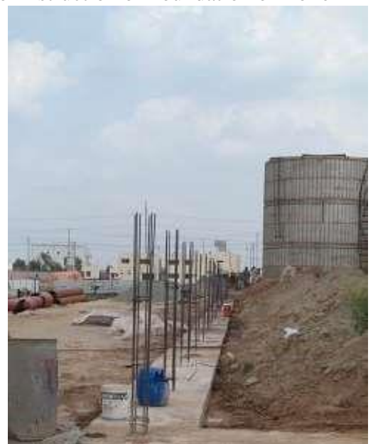
246-- Construction of Dyke Wall
