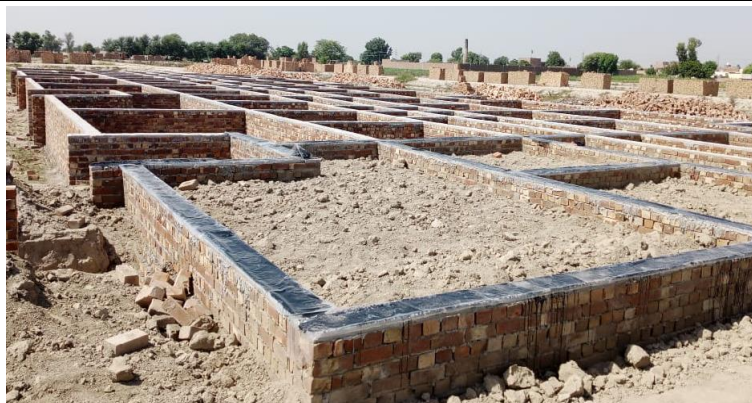
259- Construction of 714 Apartments New Depalpur City
