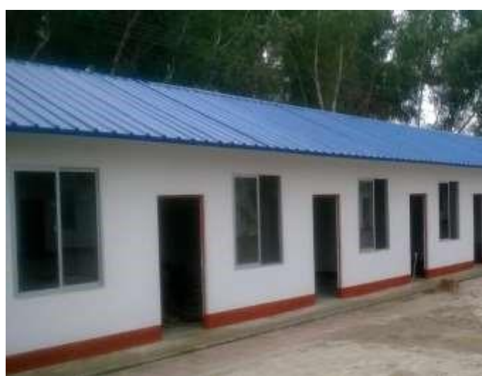
172-Construction of Chines Camp at T-4 Tarbela.
