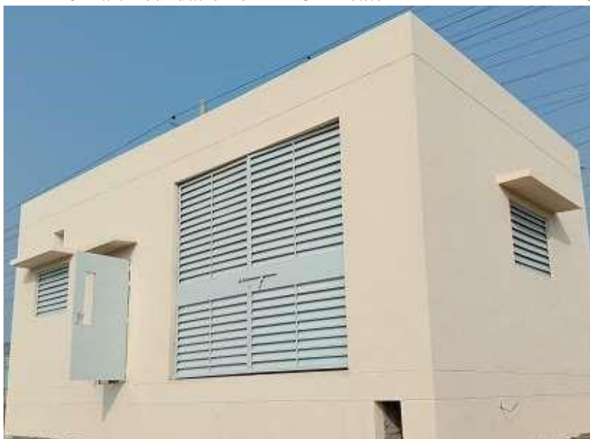
246-Construction of FESCO Room for 2500 KVA Transformer
