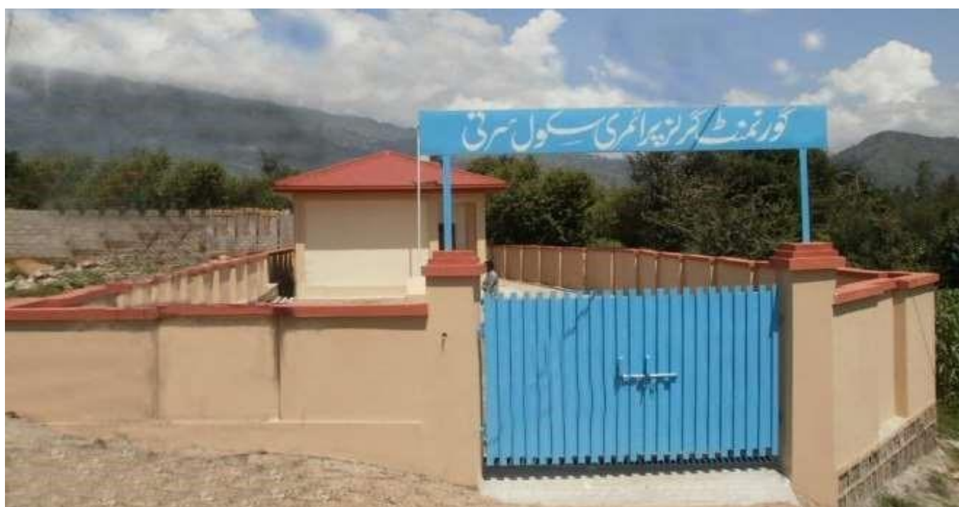
118-Completed Picture of GGPS Sarni UC Phullran, District Mansehra.
