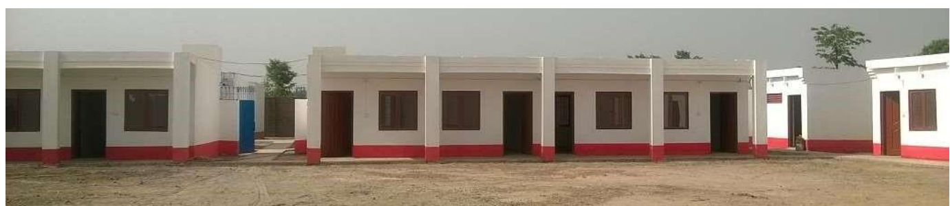
204-205-Chines Camp 2 & 3, Division – II, KLM-III Project of CR20G
