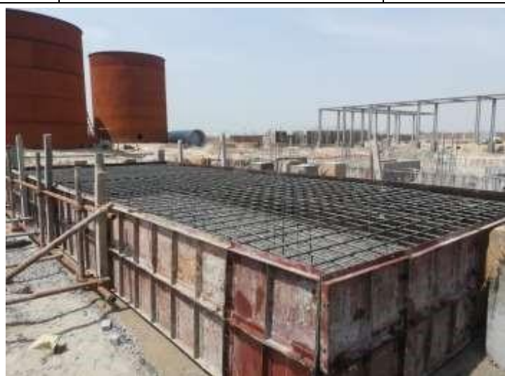
246-Raft of Machine Foundation of Boiler
