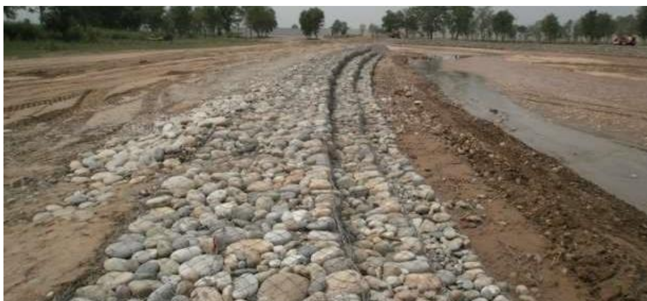
131- Repairs of Surat Nullah at New Escape Electric Power Project Mangla.
