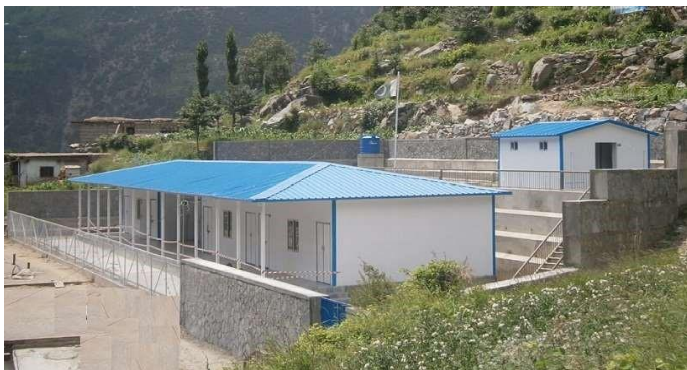
176-Construction of GPS Ghund Patay, UC Mankial District, Swat, KPK
