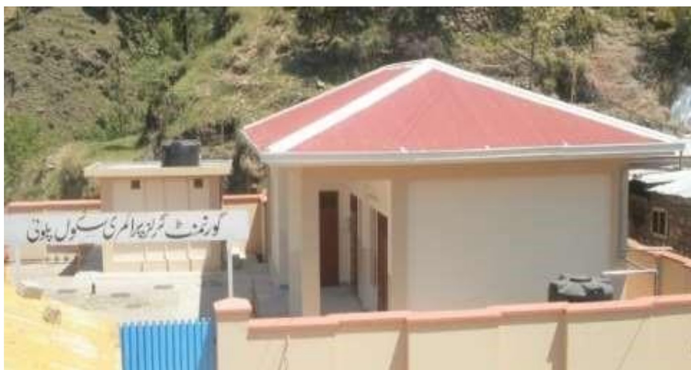
109-Completed Picture of GGPS Paloi, UC Jabori, District Mansehra.
