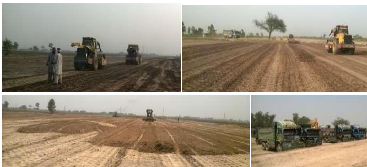
207-213-Earthwork for Road Sub-Grade at Division-II, KLM-III KM 1127 ~ 1137
