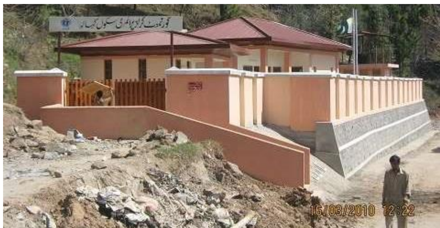
96-Completed Picture of GGPS Kahala, UC Jhandgran, District Muzaffarabad, AJK.
